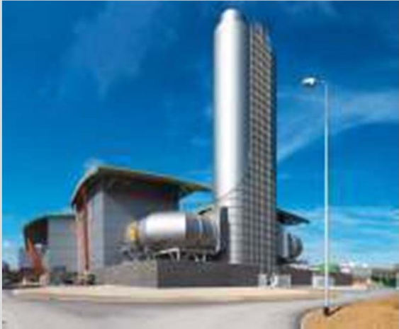
Combined cycle plant
